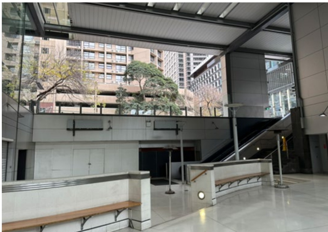
Figure 8 | View of lower ground floor, looking towards Castlereagh Street
